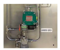
Permanent labelling, including drawing inside enclosure for future identification and maintenance
