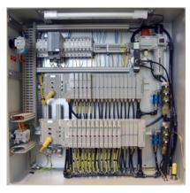
Innovative products including ultrahigh-flow directional control valves, fieldbus electronics, and modular air preparation products
