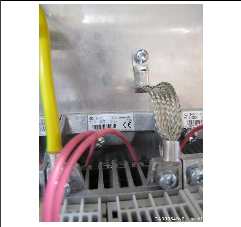
Fig. 6-26: Grounding strip between heat sink and mounting surface (example)
